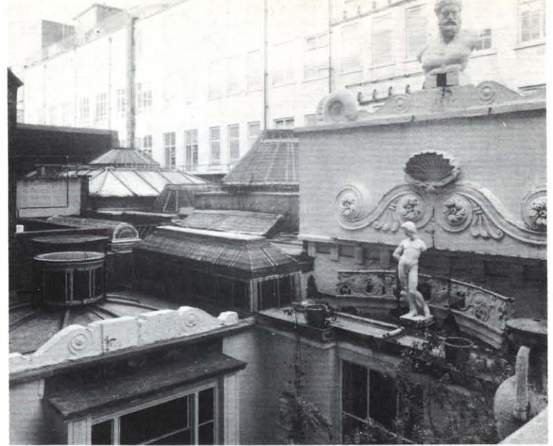
Cubierta y lucernarios del museo de Sir John Soane Ceilings and skylights of the Sir John Soane's Museum Foto: Michael Nicholson
