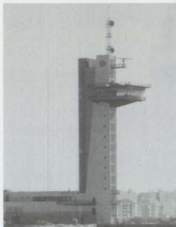
The metal window frames will be aluminum with a matt reddish finish. The remaining metal elements on the building's facade will be red coated. The glass used throughout the building facade will be smoky, specially around the Control room.
