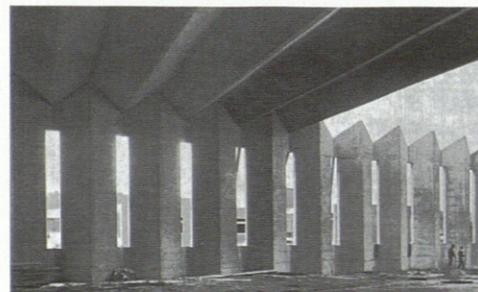
straight longitudinal bars could be used thanks to this somewhat unusual arrangement. Indeed, the National Building Service recommendation in force at the time called for only 3 layers; while this would have allowed for a thinner shell, the use of arched bars as the main reinforcement that this solution entailed was not cost-effective in this case.
