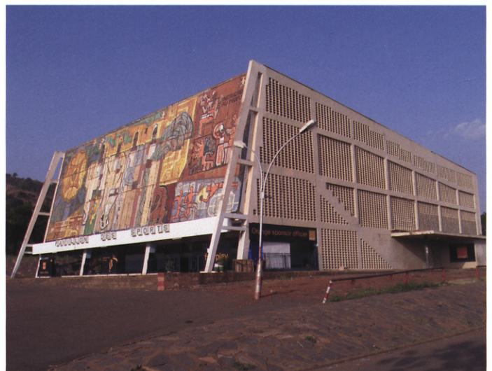
Polideportivo y piscina Modibo Keita. Sports center and swimming pool Modibo Keita.
