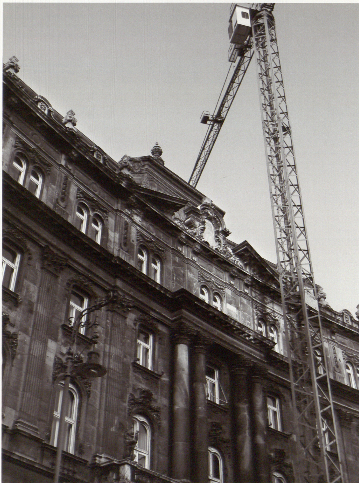
Edificio en rehabilitación en la plaza Szabadsag. A building during its restoration in Szabadsag square.
