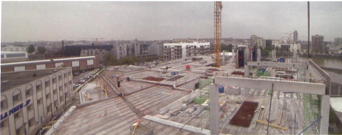
La estructura de hormigón pretensado prefabricado ajusta su geometría al solar. Éste se ubica en la ribera del Loira, próximo a zonas de equipamiento. The structure of prefabricated pre-stressed concrete adapts its geometry to the plot of land. The latter is located on the bank of River Loire, nearby to equipment areas.
