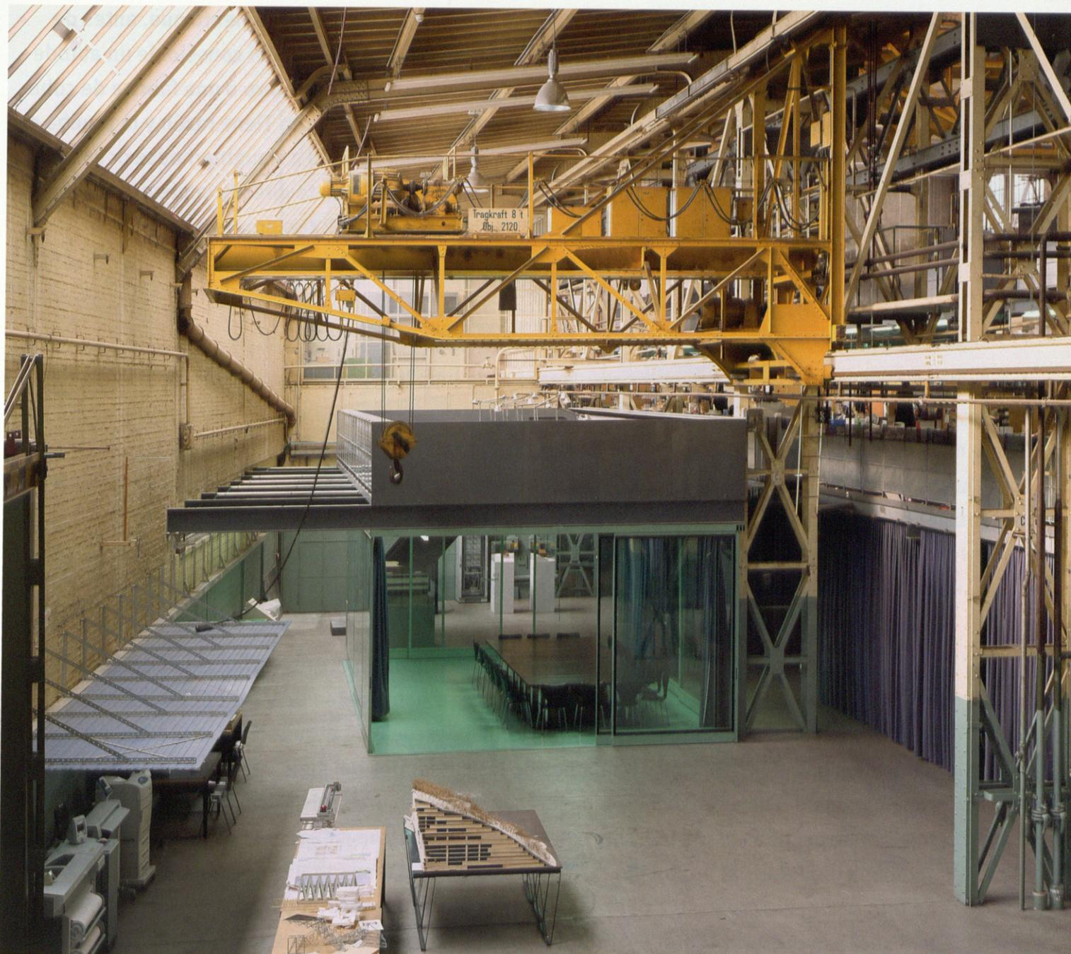
In an attempt to avoid the modification of the structure of the former workshops, different steel platforms have been made. The areas released on the ground floor have been used for the library, auditorium and school work areas. Partial reformatations, area extensions or attachments of nearby buildings have been carried out as the use of the building required so. Although the initial plans of 1991 were only for five years, different renovations were authorised in 1997 and 2003.
